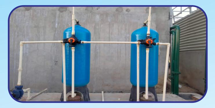
ACF performs the important duty of eliminating foul smelling gases e.g. Hydrogen Sulphide, Carbon Dioxide etc. It also establishes normal color of water.
