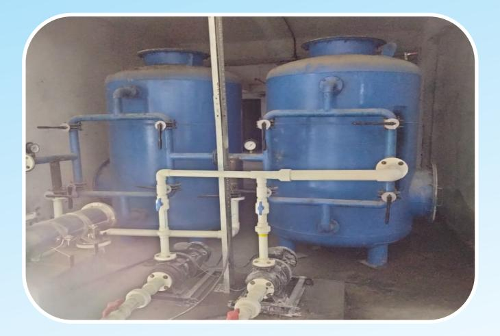
Sand of various sizes and varieties coupled with gravel and brick blast plays important role in water purification. At times upper layer may have to be partially replaced after use. It refreshes the sand filter for fine working.
